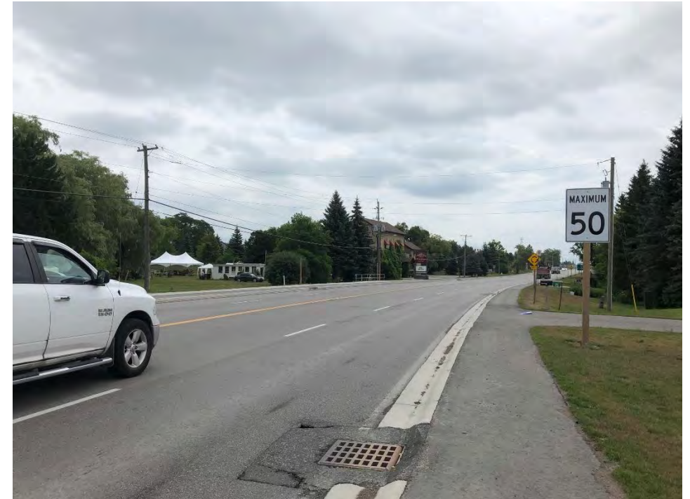
Wellington Road 46, Aberfoyle
